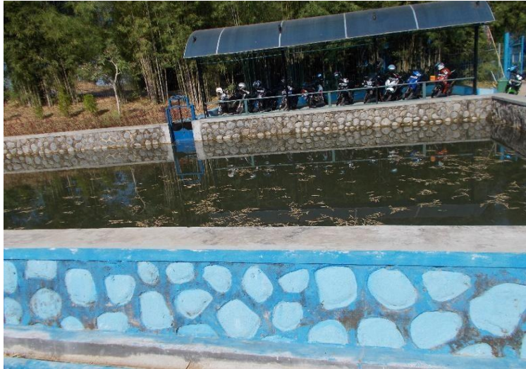
Gambar 3.11 Unit Prasedimentasi PDAM Intan Banjar
