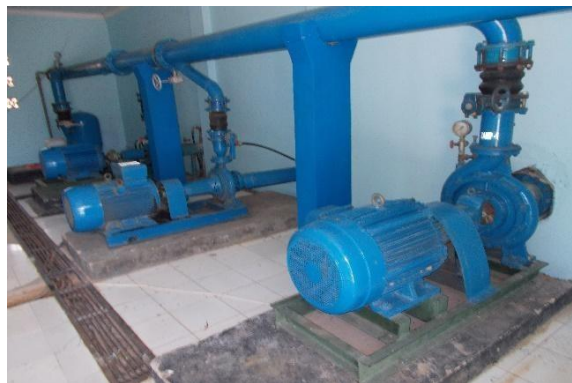
Gambar 3.5 Pompa Distribusi IPA Pinus
