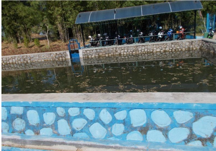
Gambar 3.11 Unit Prasedimentasi PDAM Intan Banjar
